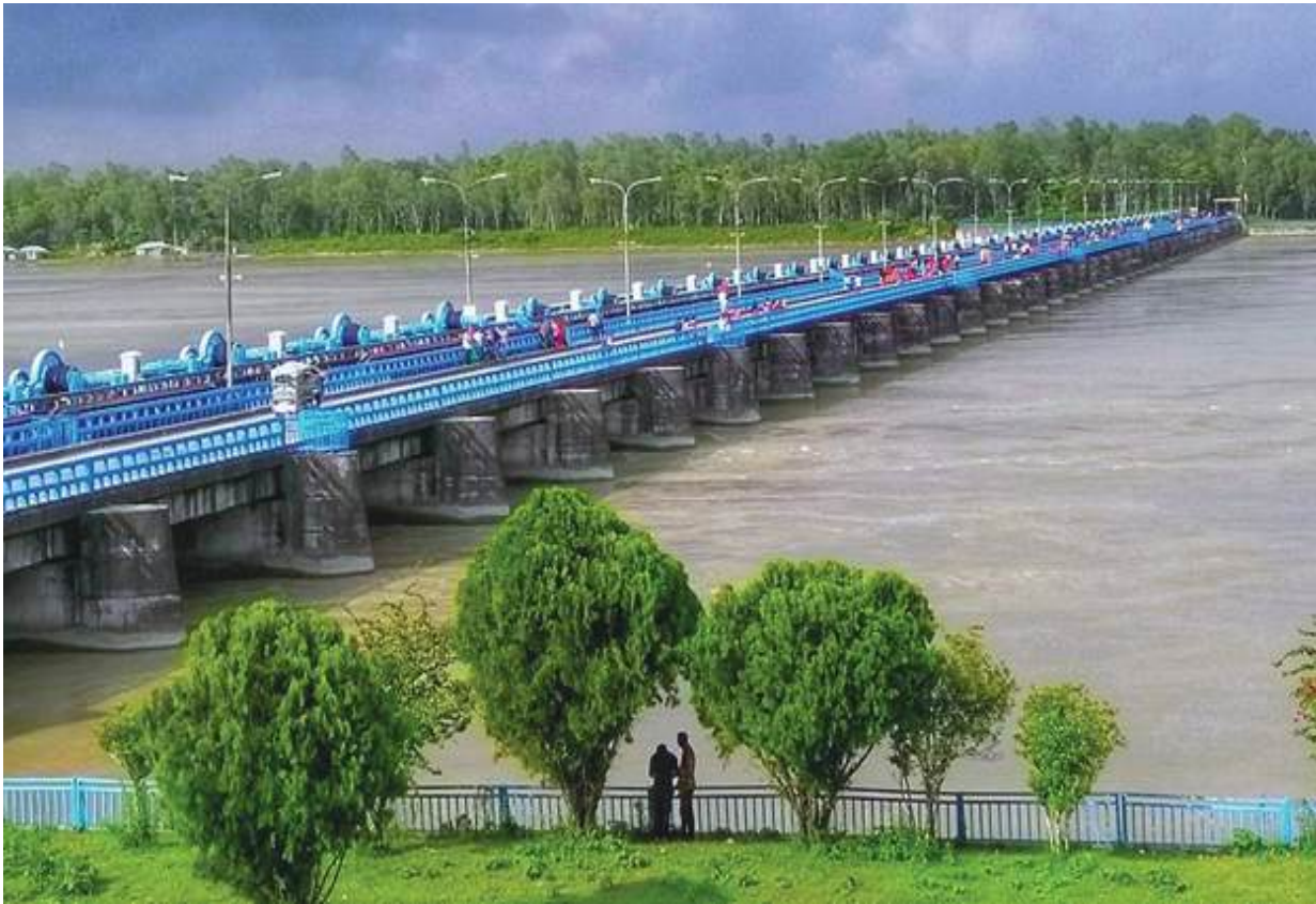
Teesta Barrage (Credit: Masnad, CC BY-SA 4.0 < https://creativecommons.org/licenses/by-sa/4.0/ >, via Wikimedia Commons)
